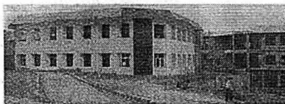
The white portion is OPD which has become functional
